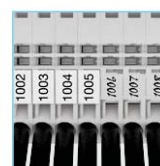
Clear terminal block identification Top large marker. Hand pre-marking before final marker installation
